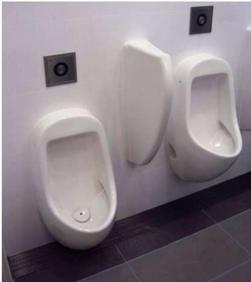
Illustration 11: Adult height and child height urinals, stainless steel grating over drainage
