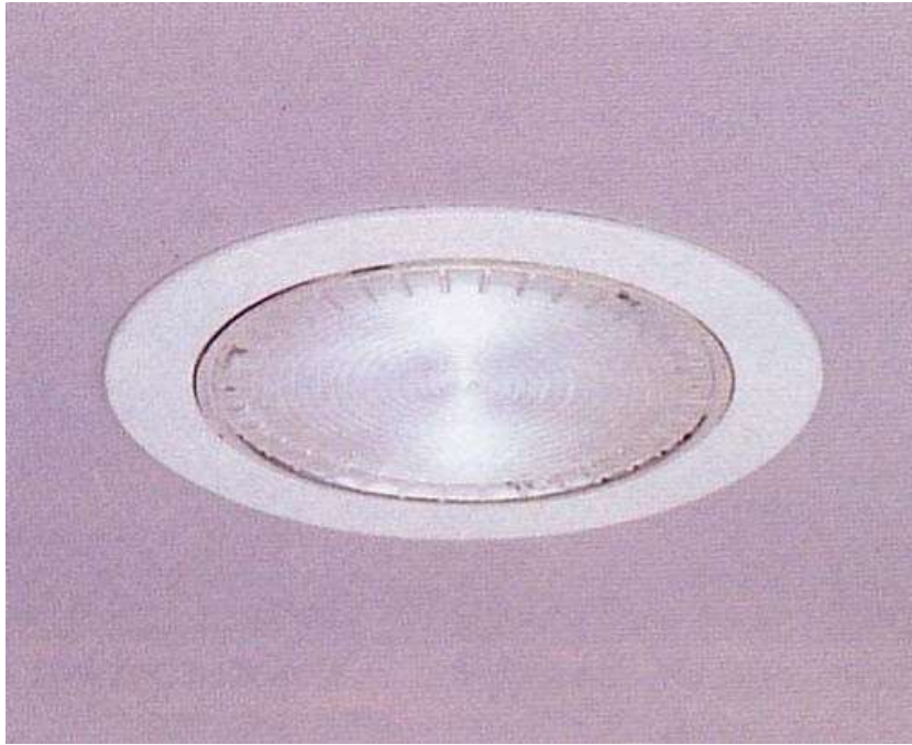
Illustration 7: Non-suspended PLC downlight, mounted onto ceiling
