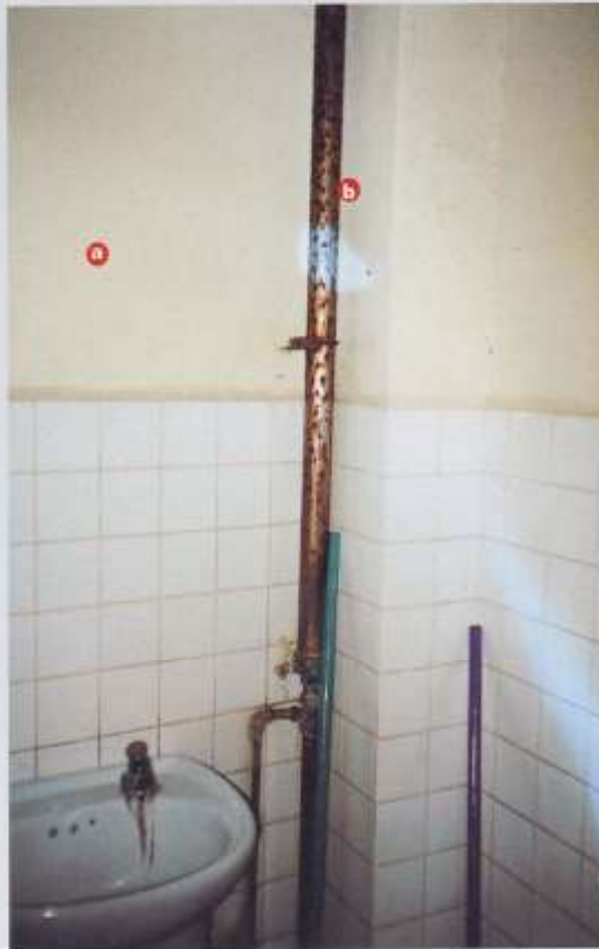
a. Painted Surface b. Exposed Piping
