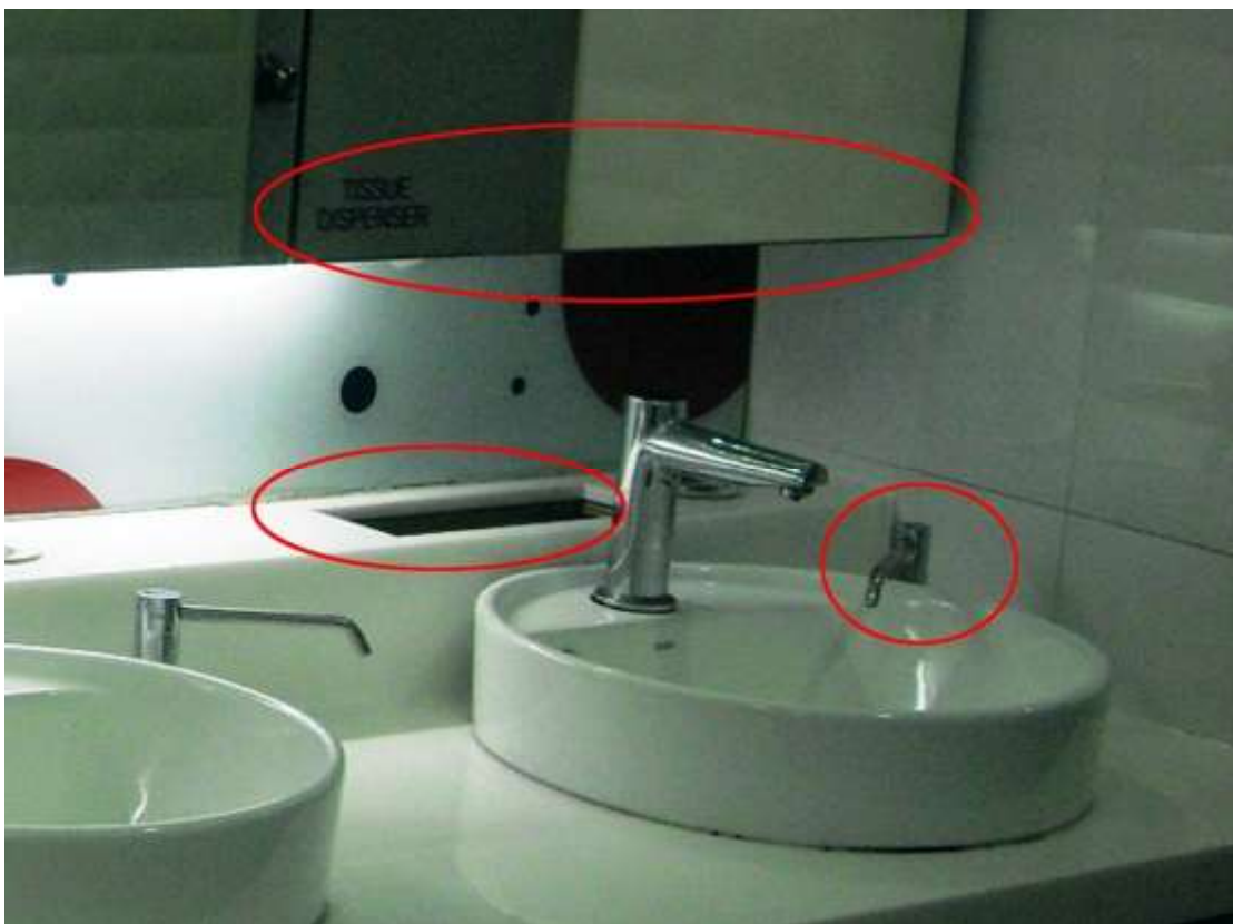
Illustration 16: One-stop provision of auto sensor tap, soap dispenser, litter bin and paper towel dispenser or electronic hand-dryer at wash basin area.
