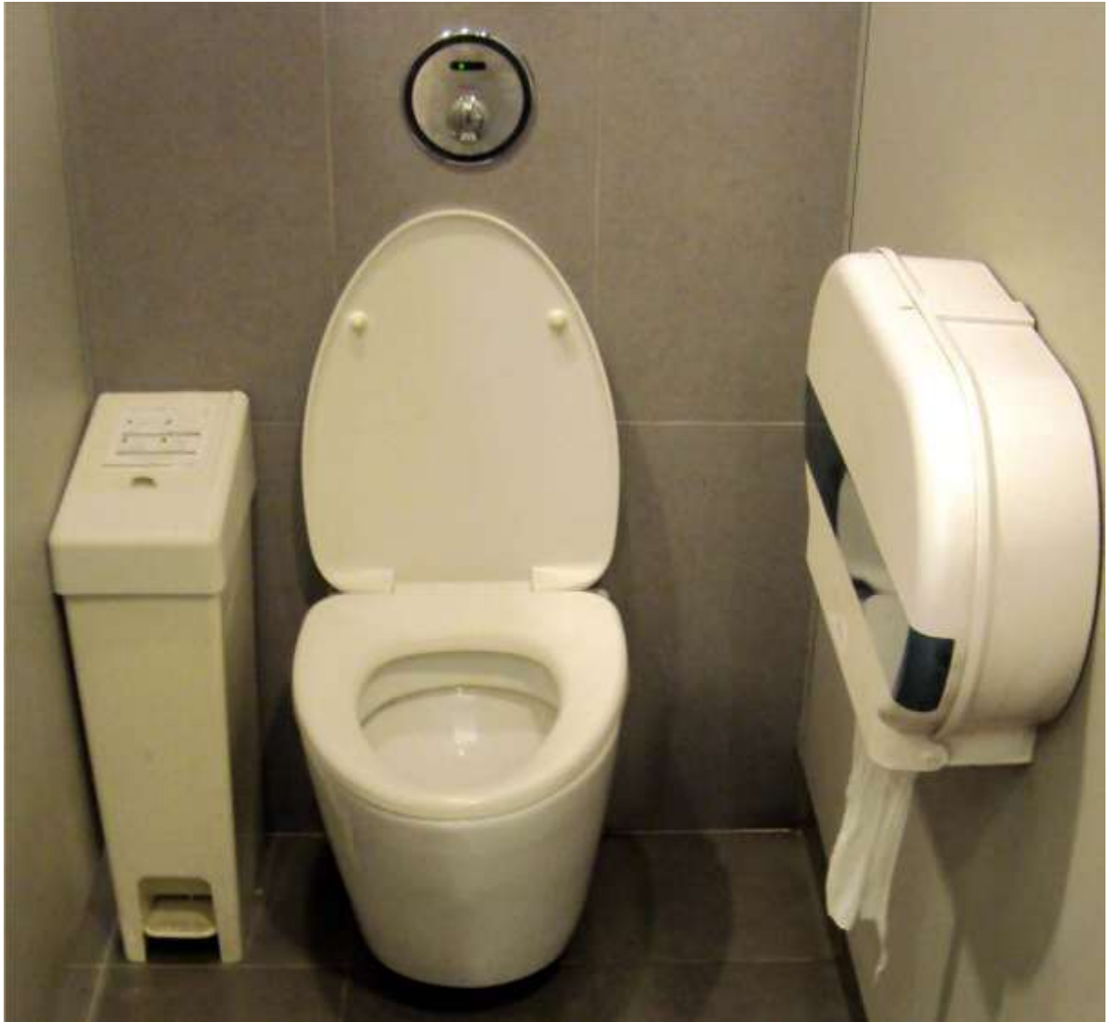
Illustration 17: Wall hung WC with double-roll toilet paper dispenser and foot operated sanitary bin
