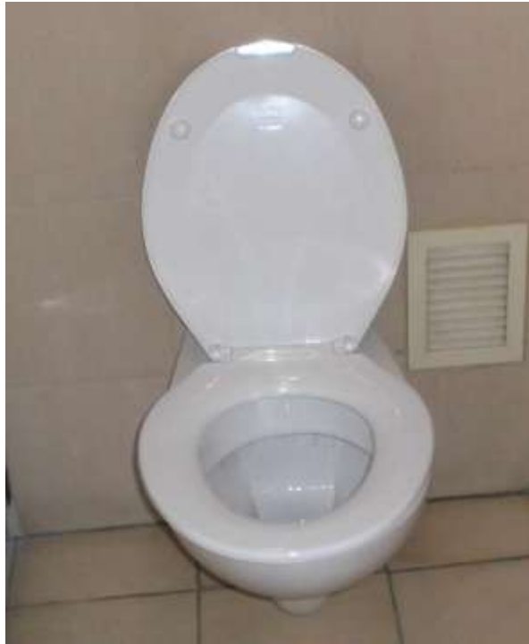
Illustration 24: Low level mechanical exhaust
